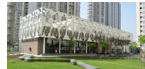
Facade structure made of TRC © Raina Industries Pvt. Ltd
