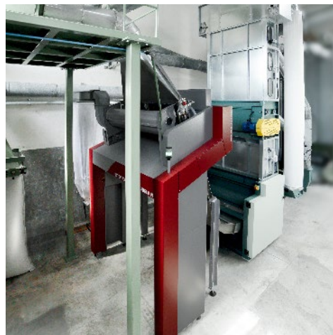
UJVSN installation in nonwovens production © 2022 USTER
