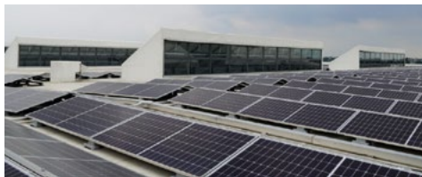
The new production site generates its own electricity through solar panels on the rooftop © 2023 Trützschler
