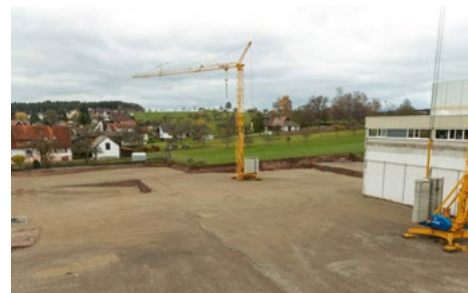
The construction ground of the new TCC site © 2023 Trützschler
