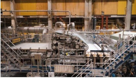
Production hall in Renewcell's textile recycling facility Renewcell 1 in Sundsvall © 2023 Renewcell
